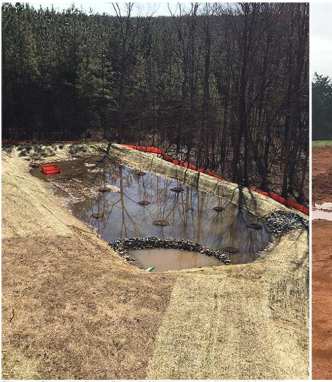
Figure 7. Example of compliance (left) and noncompliance (right) with erosion and sediment control requirements. Photos courtesy Berkley Group.
